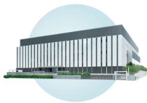
QTnet Fukuoka Data Center 2
