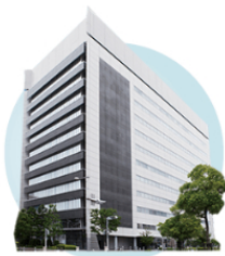
QTnet Fukuoka Data Center 1
